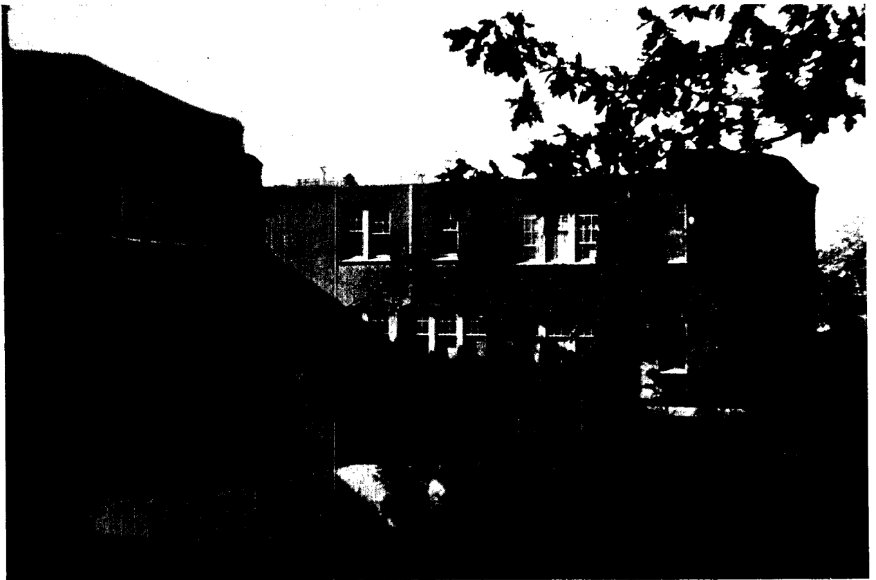
APPLIED SCIENCE BUILDING
