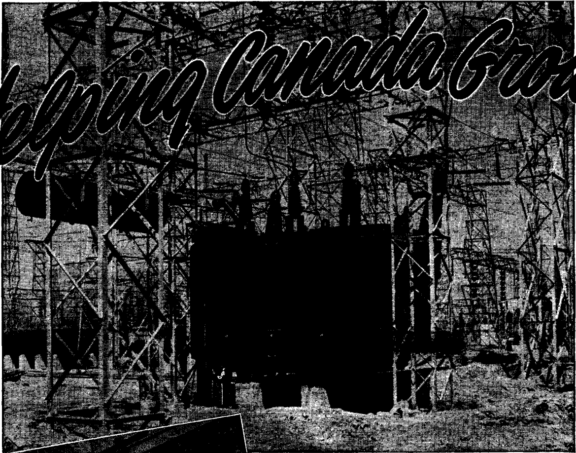
Canada's largest transformer—one of eight rated 90,000 kva built by Canadian General Electric for the HEPC of Ontario. Their large size is evident when compared with the man standing at the lower left-hand side.
