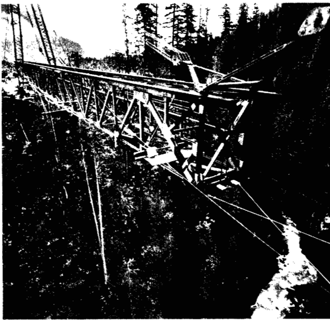
Launching the 102-metre main truss of a bridge over Pashleth Creek, B.C. The bridge will carry 235 tonne off-highway logging trucks over the steep canyon. Design and supervision by Buckland and Taylor Ltd.
