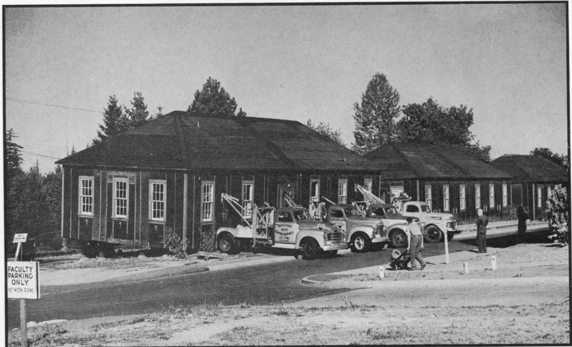
Moving Army Huts into place on the Campus—a common scene in the early post-war years, 1945-1947.
