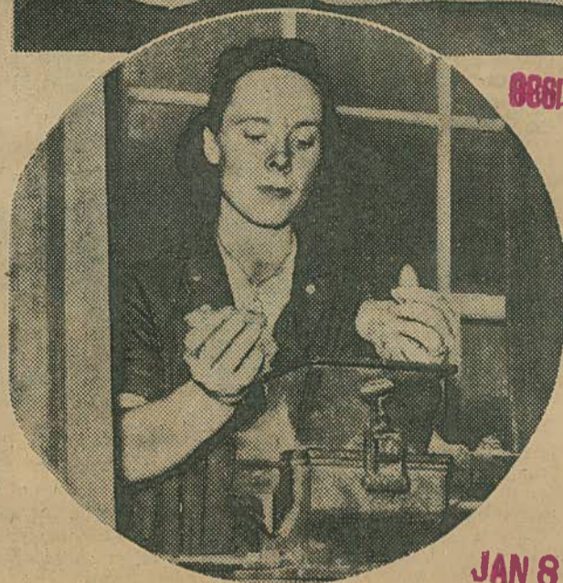
Right below—Miss Norma King is studying towards her master's degree in geology, but she also takes courses in mining engineering. Unassisted she runs samples of B. C. nickel through an ore crushing machine and does her laboratory work for a course in ore dressing.
