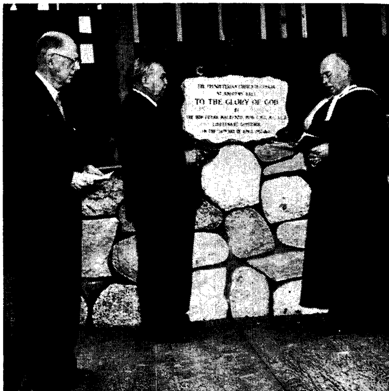
Lieut.-Gov. Frank M. Ross (centre) declares "This stone well and truly laid" at laying of foundation stone of St. Andrew's Hall, $240,000 Presbyterian College under construction at UBC. Presbyterian Moderator R.S.M. Kennedy (right) gave prayer of dedication. Mr. Justice A. M. Manson (left) organized fund-raising committee.
