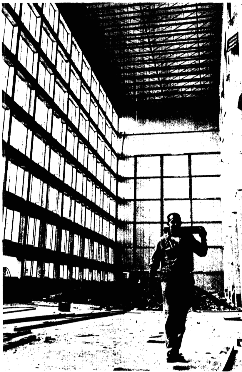
CONSTRUCTION WORKER Gordon Valough strides across empty space at the rear of UBC's library, currently being filled in to provide additional stack space, reading room accommodation, and private reading and study cubicles. An additional 44,000 square feet of floor space will be added to the library, and shelf space increased to provide for a total of 1,000,000 books. Total cost of the project, which includes other interior improvements to simplify library organization, is $866,500. Architects are Toby, Russell and Buckwell. Photo by Brian Kent, Vancouver Sun.
