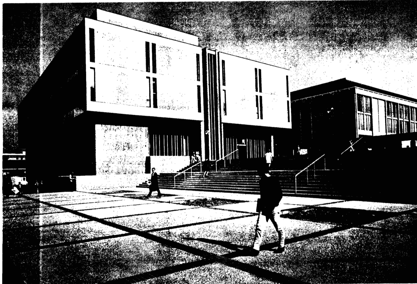
NEW MUSIC BUILDING at UBC is the latest addition to the Norman MacKenzie Centre for Fine Arts. Located adjacent to the Frederic Lasserre building, seen at right, the new music building will accommodate 300 students and contains
