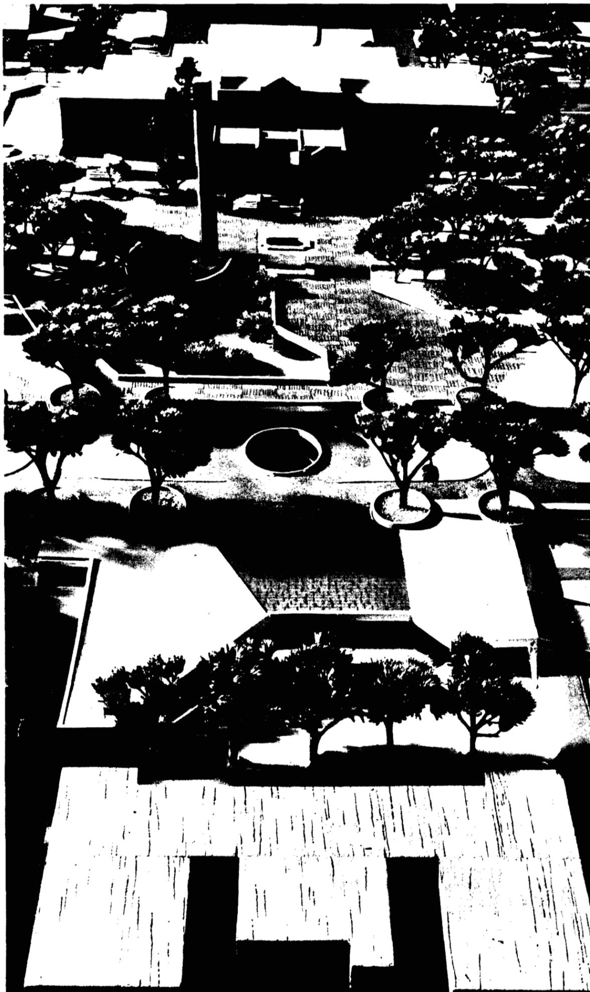
MODEL shows how the new Sedgewick Library will be located between the Main Library, top, and the mathematics building, bottom. Eight concrete caissons, enclosing the roots of existing trees on the Main Mall, will travel down through the two-storey building. Students on both floors will be able to look
