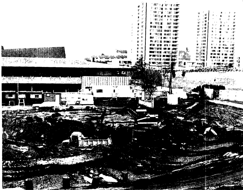
Contractor has started excavating new UBC swimming hole
