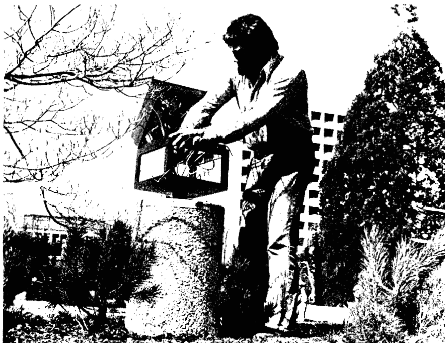
Physical Plant electrician David McCall installs fixture atop new bollard lamp, one of 25 recently put in place near Main Library as part of ongoing program to improve campus lighting. The bollard lamps are so-called because the bases resemble metal posts for securing ropes on ships and docks.
