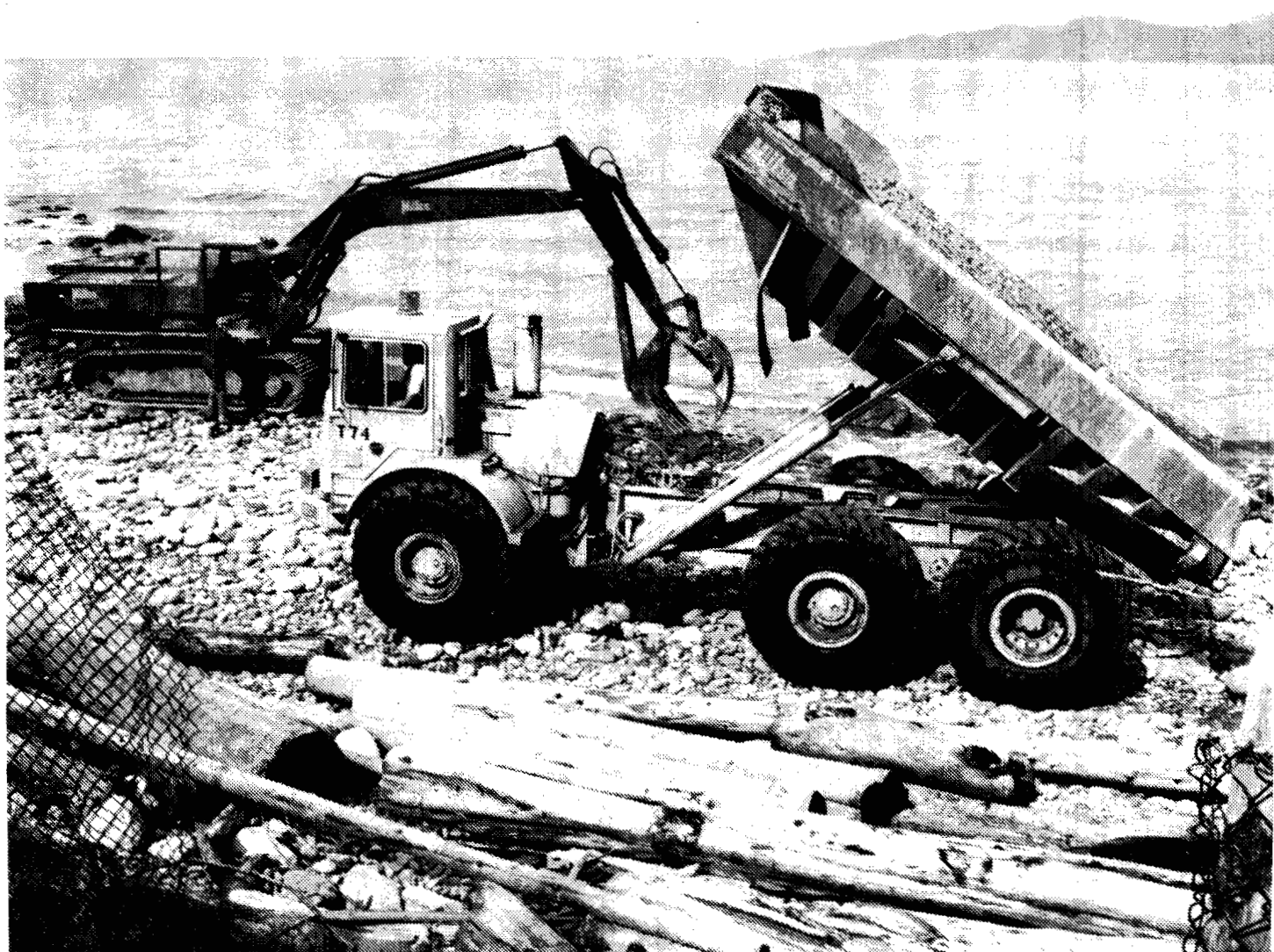
Face of Towers Beach is changing rapidly this month as work continues on construction of protective berm between the two Second World War observation towers below Museum of Anthropology.
