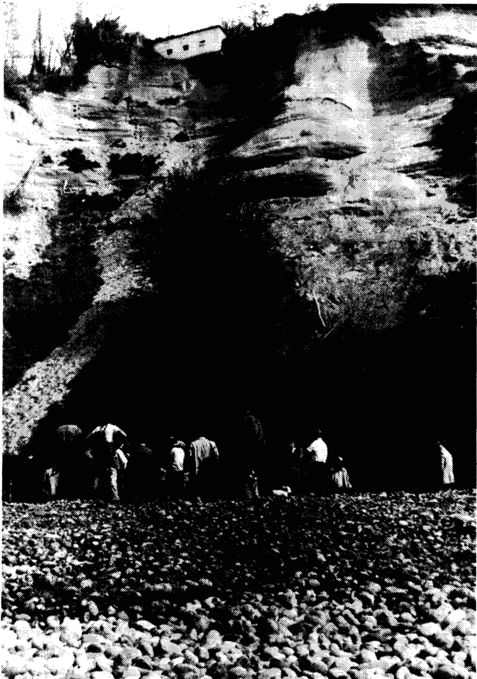
Members of Erosion Control Advisory Group toured beach on April 29 to have a look at the protective berm of rock and gravel designed to stop toe erosion of Point Grey cliff. Flat top of berm is well above high tide mark and has been covered with a foot of sand. Dune grass will be planted in the autumn. About 300 metres of beach between the two searchlight towers now is protected.
