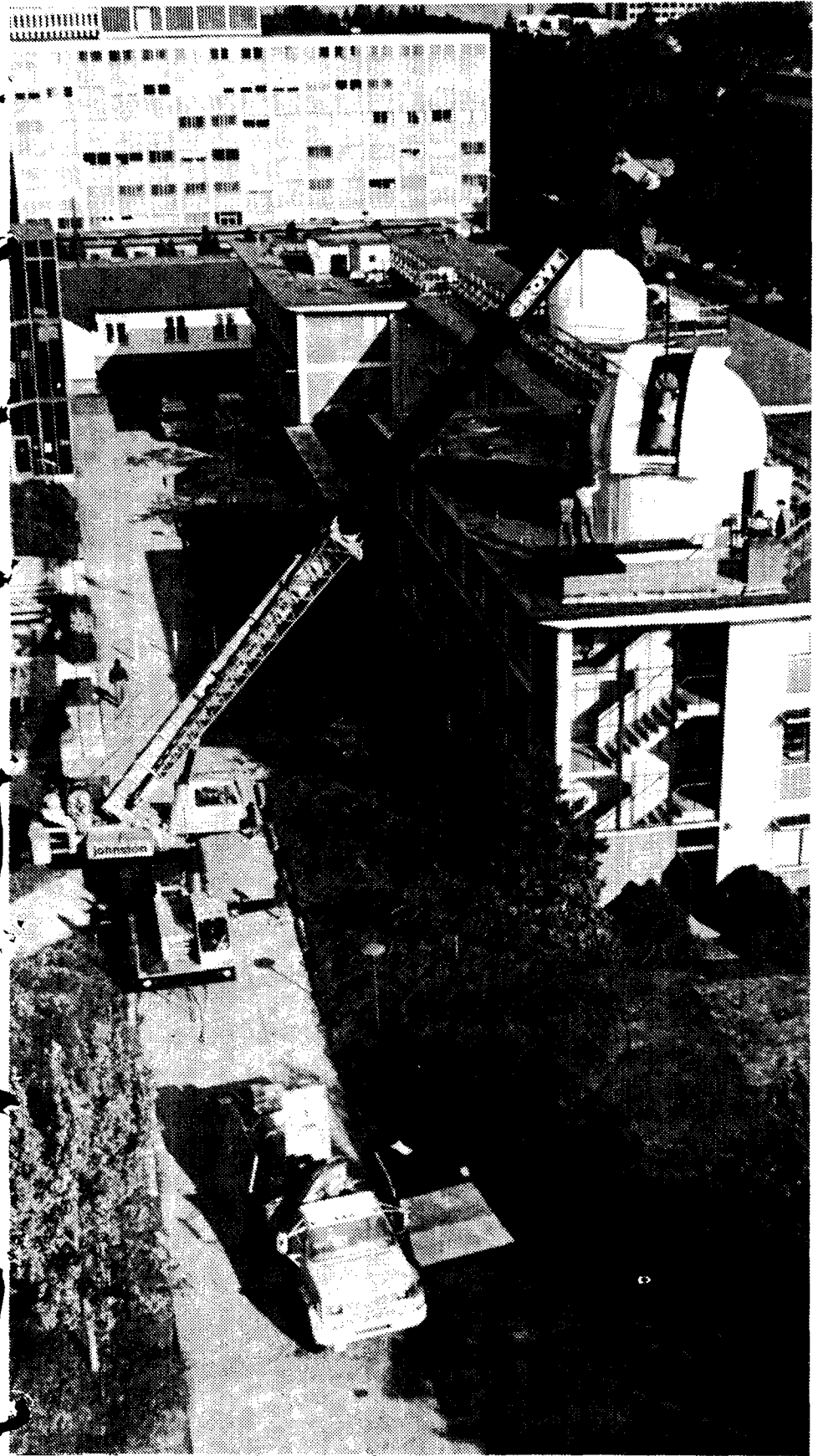
New 16-inch telescope goes into position atop Geophysics and Astronomy Building. It will be used by 4th year and grad students, and will be open for public use two nights a week starting at the end of October.
