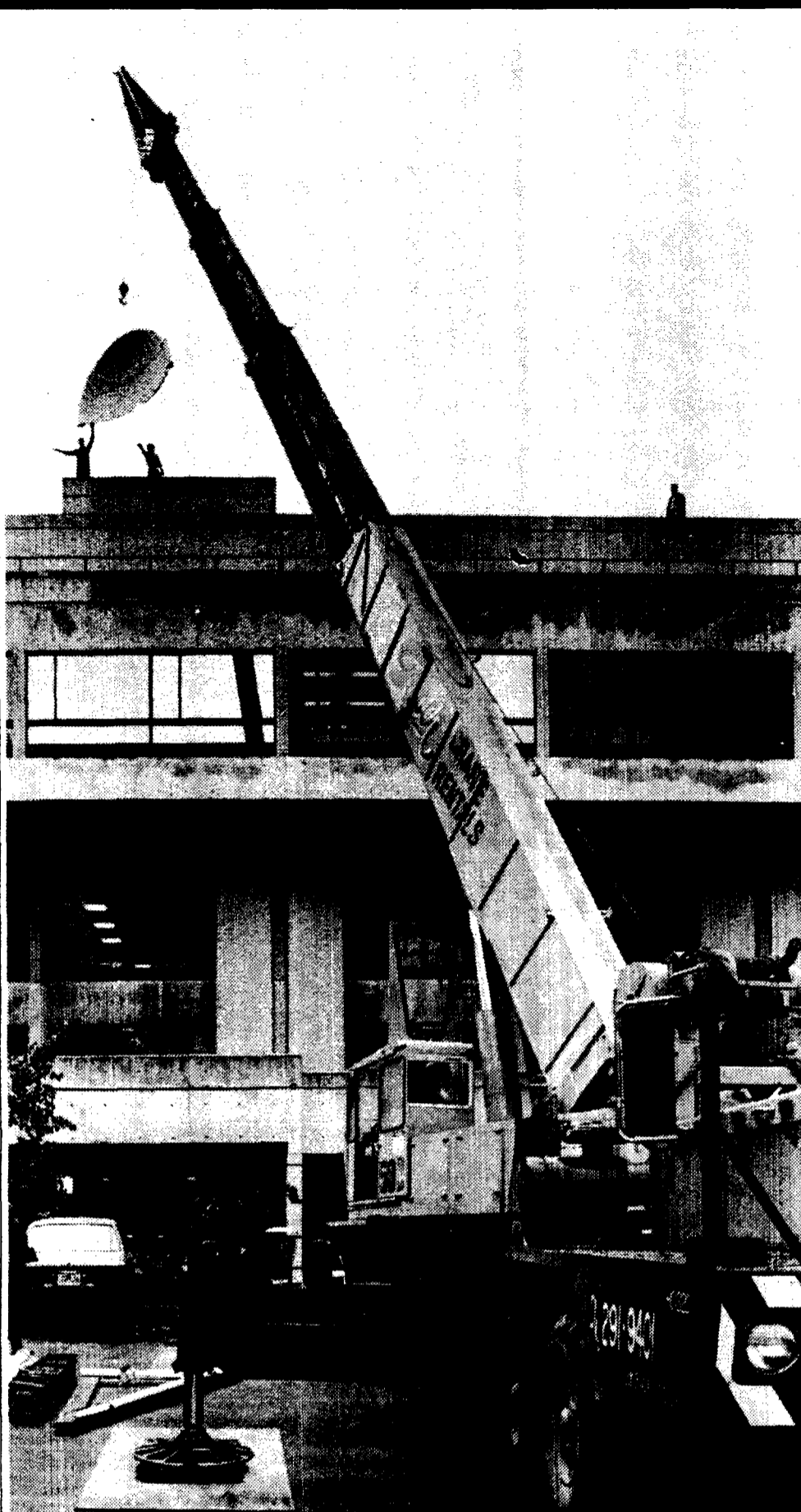
Ninety-eight hours of public educational television are now being beamed to all parts of B.C. weekly via the transmitter of the Knowledge Network, which moved its operations centre to the UBC campus last week. Giant crane, above, hoisted transmitter components to the top of the Woodward Instructional Resources Centre, linking UBC with 53 B.C. communities who receive programs via satellite earth stations or cablevision. Fall program guides are available from network's UBC offices in the Library Processing Centre, 224-6511.
