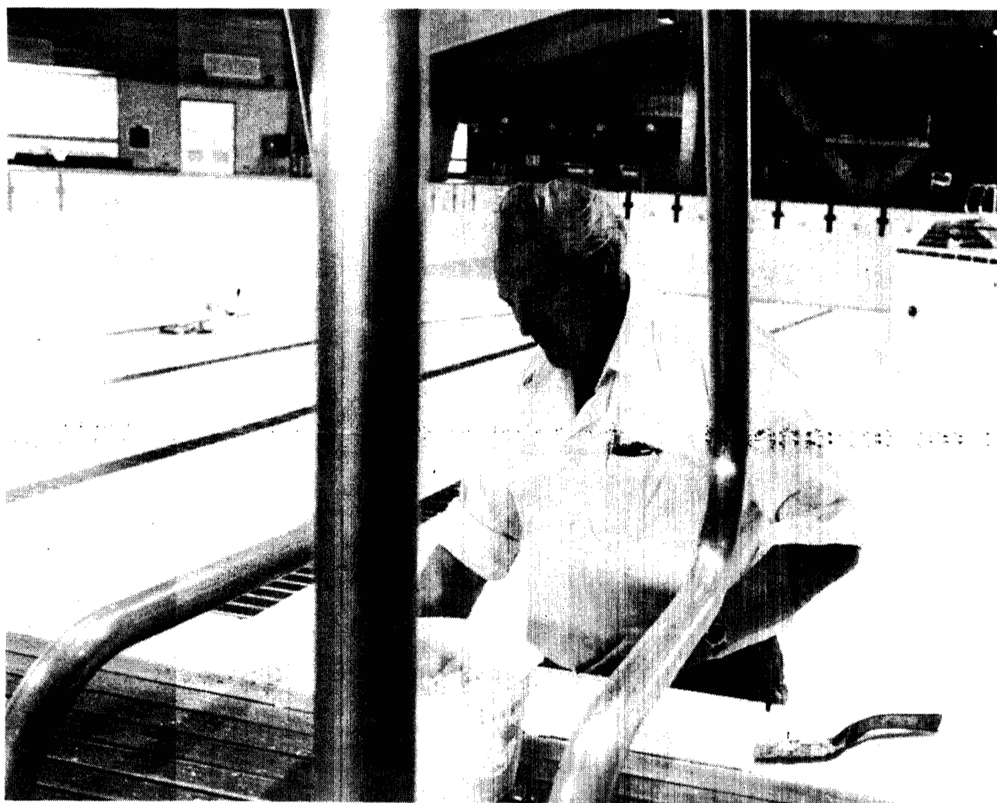
Physical Plant mason Hank Hoppmann is one of the few people at UBC who can claim that he's had the covered pool of UBC's Aquatic Centre all to himself. But not for swimming. Hank and other maintenance workers are currently putting the indoor pool in tip top shape for its June 21 reopening. Hank is going over the pool foot by foot and regrouting tiles. In the meantime, the outdoor pool at the Aquatic Centre, which has just undergone an $886,000 facelift, is open for business daily.
