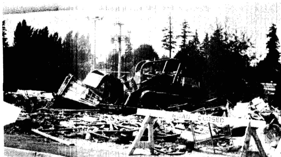
Gone is this hut on West Mall, one of three demolished last week on the site of the new Physical Plant building. The former army huts are among the oldest on campus, brought to UBC in 1945 and 1946 for use as classrooms and offices. The huts' most recent occupants, members of the oceanography department, have moved to quarters in the new Bookstore building.
