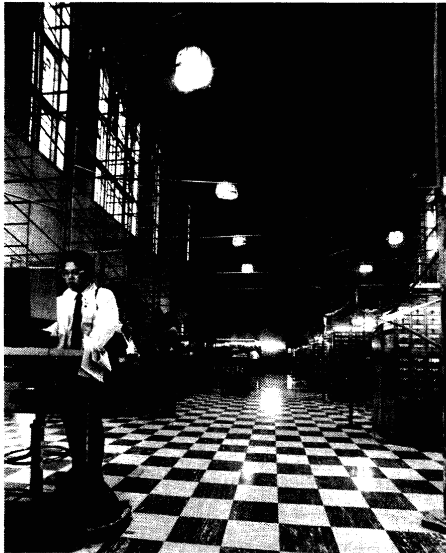
If you're looking for a quiet place to study this winter, avoid Main Library. The normally hushed atmosphere of the library will be disturbed for several months as workmen install a new sprinkler system to bring the building up to fire safety standards.
