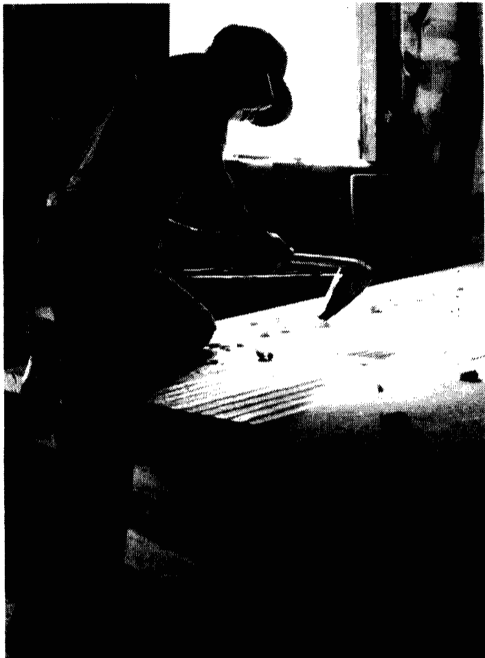
A Haida artisan adds texture to a cedar wall, part of a longhouse being constructed in Masset on the Queen Charlotte Islands for the new National Museum of Civilization in Ottawa. Work on six longhouses -- one from each of the major cultural groups of the Northwest Coast Indians -- will form the centrepiece of the museum's Grand Hall. The work is being subcontracted by the Museum of Anthropology.
