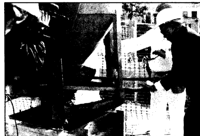
The Honourable David Lam presides over concrete-pouring ceremony at the site of the new Management Research Centre.
