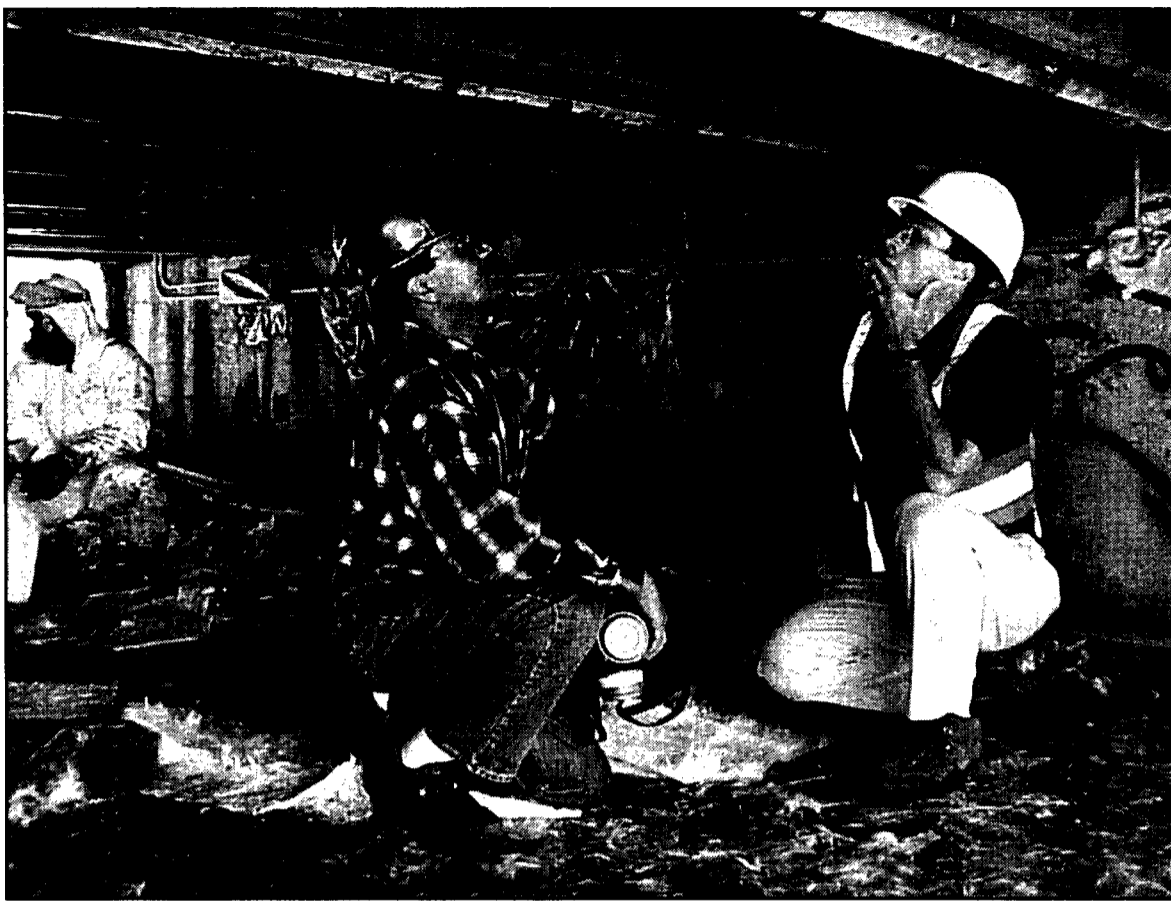
Civil Engineering Prof. Nemkumar Banthia (left) and Ian Sturrock, an engineer from the B.C. Ministry of Transportation, inspect the underside of a 46-year-old bridge near Duncan B.C. sprayed with a revolutionary fibre-reinforced polymer coating. The coating, developed by Banthia, is designed to repair and double the strength of bridge decks for half the cost of traditional repair methods. Civil Engineering Dept. photo
