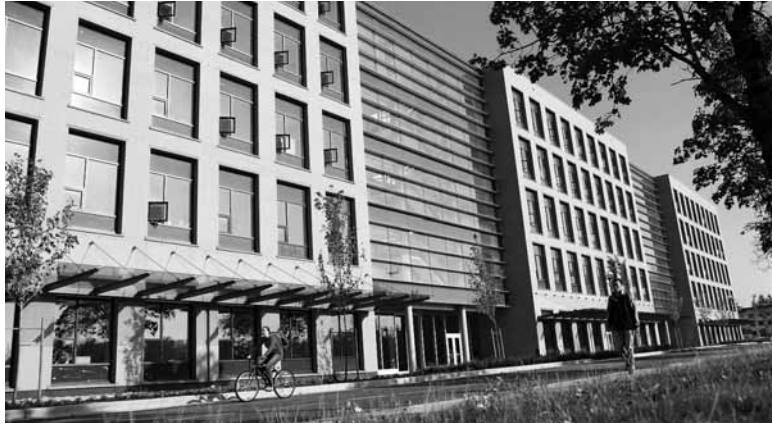
The UBC Life Sciences Centre is not only the largest building on campus, it's also one of the "greenest."
