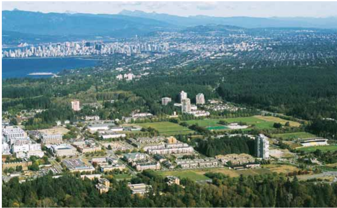
Hawthorn Place neighbourhood (above) was once the infamous Lot B parking lot. Times are a changin'; below: UBC will showcase leadership in sustainability at the World Urban Forum
