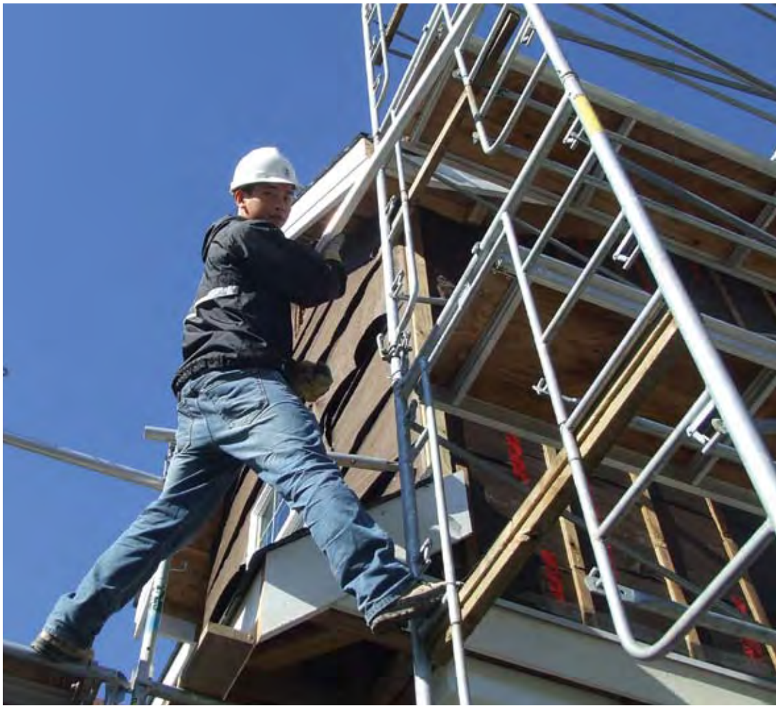
Civil Engineering student Manuel Jacinto helped build non-profit townhouses for Habitat for Humanity during 2008 Reading Week.
