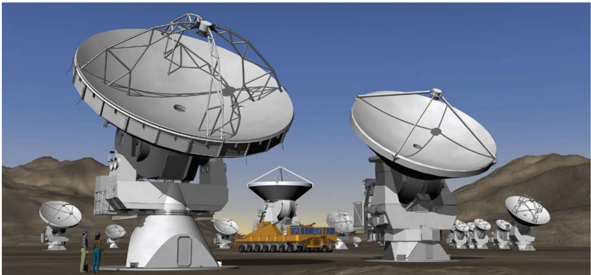
ALMA's location in the Atacama Desert is one of the highest, driest places on Earth, making it ideal for astronomical research at millimeter wavelengths, which are absorbed by atmospheric moisture.
