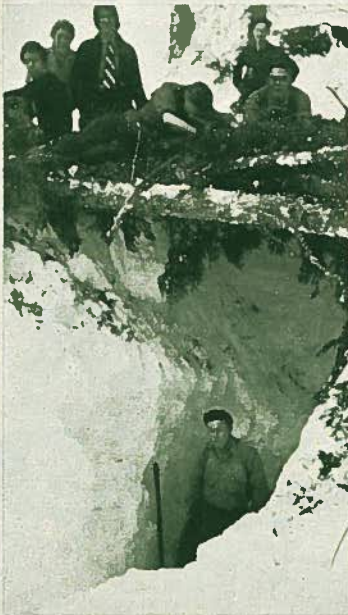
DIGGING OUT THE V.O.C. CABINS
