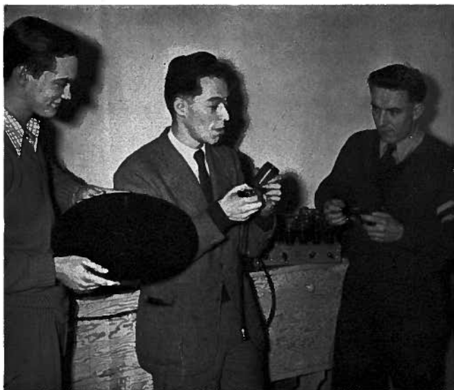
NEW CONSOLE took much time on part of engineering staff before it was ready to be installed in new control room, turntables take 16" records
