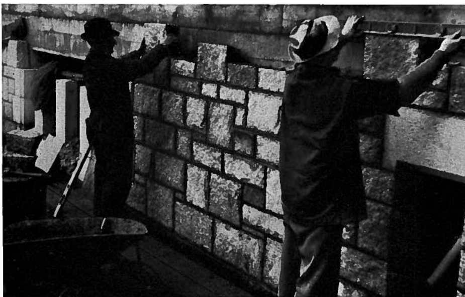
WORKMEN FUSS WITH LEVELS AND MEASUREMENTS IN APPLYING STONE FACING TO NEW LIBRARY WING.
