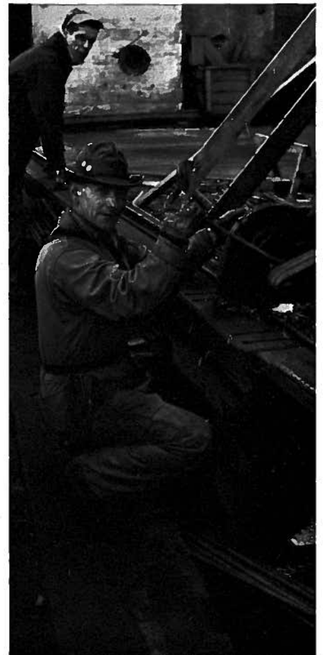
RE-INFORCING steel is cut into lengths as workmen prepare to pour concrete for Library wing
