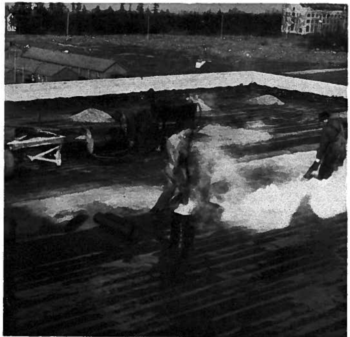
UNSEEN by most students, workmen sweatily work through heat to tar roof of the new Library wing.
