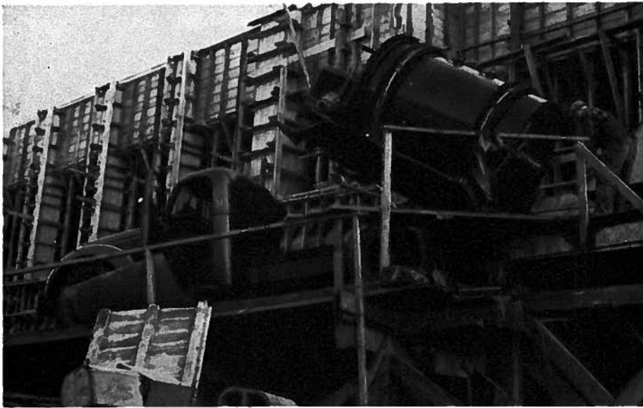
CEMENT TRUCK RUNS UP FANCY RAMP TO DUMP ITS LOAD DURING BUILDING OF NEW ENGINEERS' HOME.
