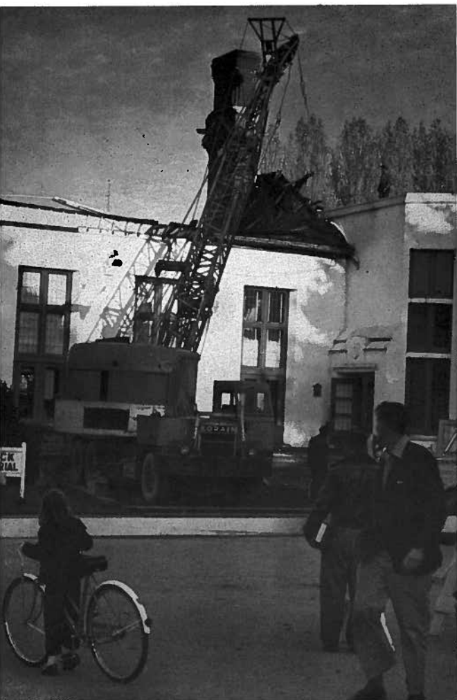
Huge crane lifts collapsed roof from the main lounge as the reconstruction of the Brock gets under way.
