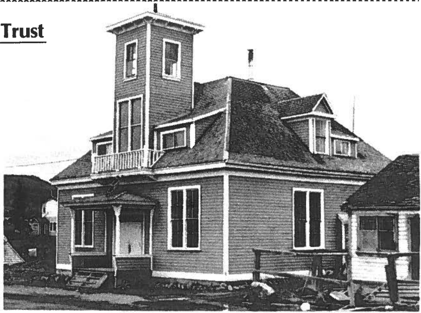
The Atlin Courthouse in 1981 before the Atlin Historical Society began its major restoration project.
