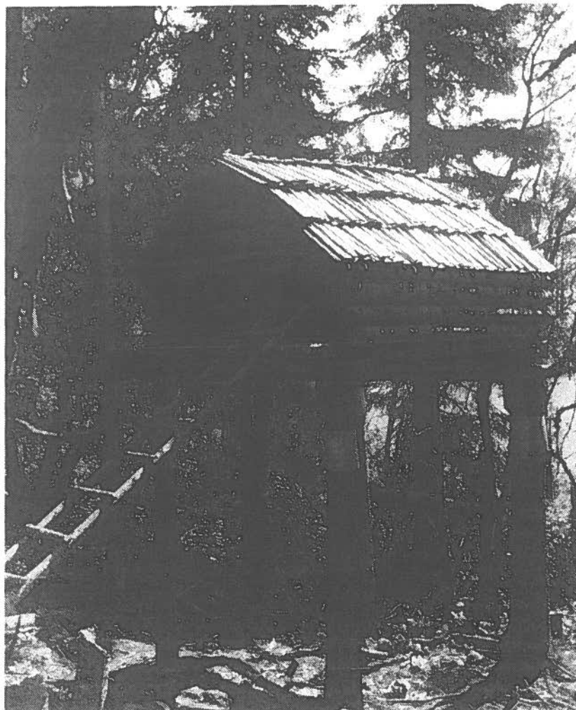
Survey party's storehouse constructed at Bowser Lake, September 1950. The metal attached to the tree trunks helped keep out marauding animals.
