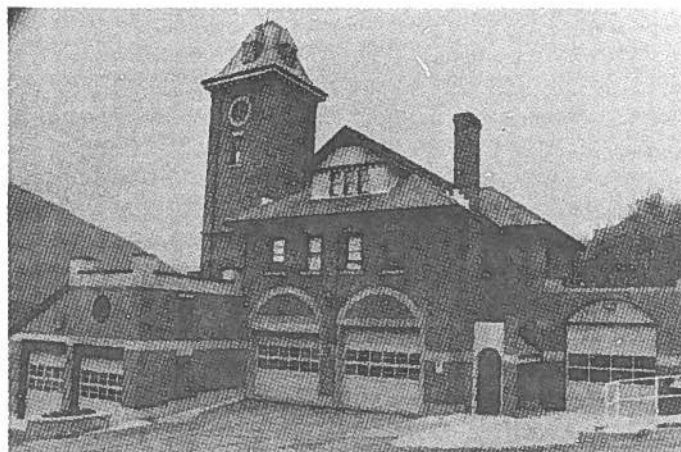
Nelson Firehall, 1912-13. Originally the horses used to pull the fire wagons were stabled in the rear. Although slightly modified to accommodate motorized vehicles, it remains a functional design combining fire and life saving services with features of the Italianate Villa style.
