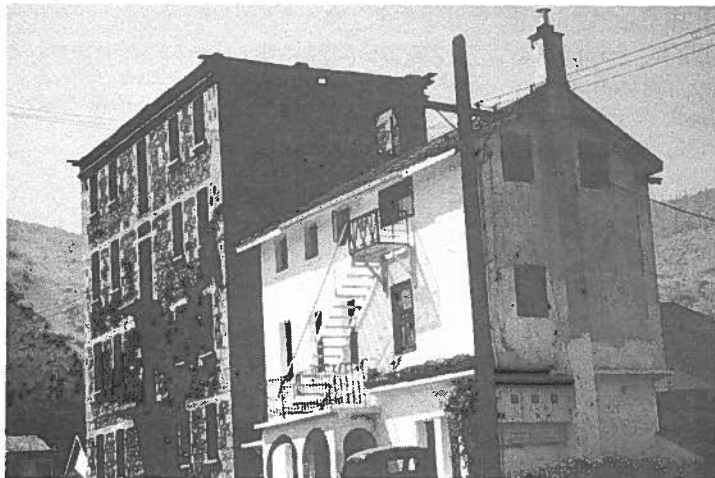
The Stone Castle and Residence, East Trail, B.C. This was taken in 1966 before complete finishing.
