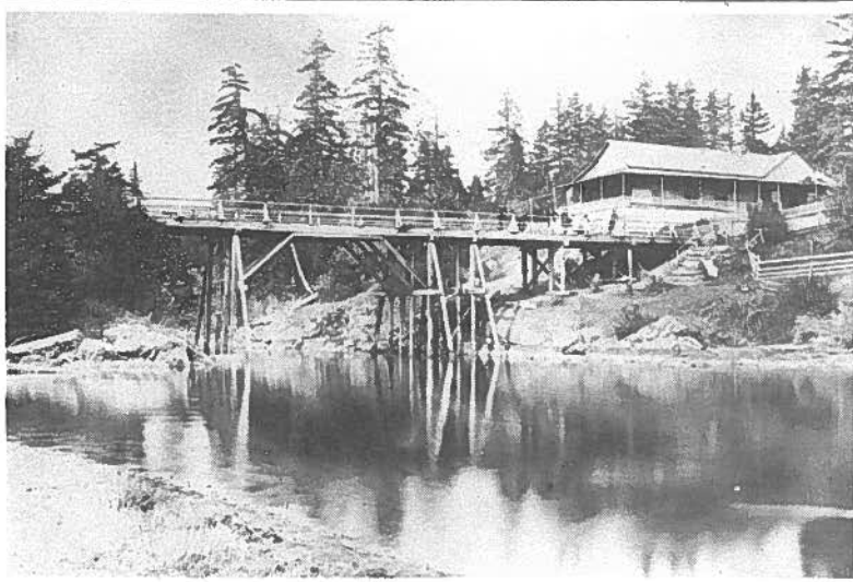
Parsons' Bridge, Victoria, prior to 1900 (now on Hwy 1A). This crosses Millstream where it enters Esquimalt harbour. The building was an inn and is now the location of Six-Mile Pub. This timber trestle was originally built in 1873 and subsequently upgraded to two two-lane curved concrete bridges. Photo courtesy of BCARS C#8030 N# F-9390.
