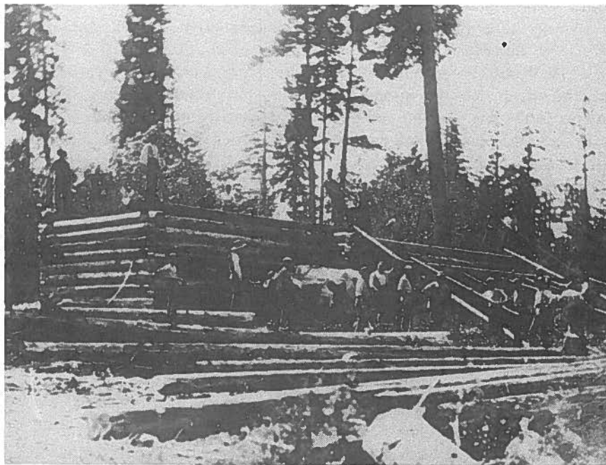
A work bee to build St. Anne's, June 24, 1894. Note the "corner" men standing atop the logs. They are R.P. Wallis, J. Lowery, James Dunn, Otto Renz, W. Cheney, W. McKenzie, B. Harris and J. McKinnon, carpenter in charge. Others shown are W. Mills, I.G. Davis, A. Crump, D.A. McMillan, W.H. Lee, A.N. Hirst, A. Cotton, H.R. Lee, W. Groffin and J. Craig.
