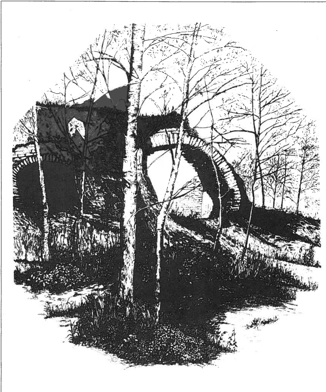
Two coke ovens at Hosmer, as seen in 1980 by artist Sandy Lightfoot, show that time has moved the insulating dirt from atop the brick ovens and spread it across what was a level wharf or walkway. When operational, a hopper car called a "Larry" ran on tracks above the ovens. The Larry was equipped to load both the east-facing and west-facing ovens standing back to back.
