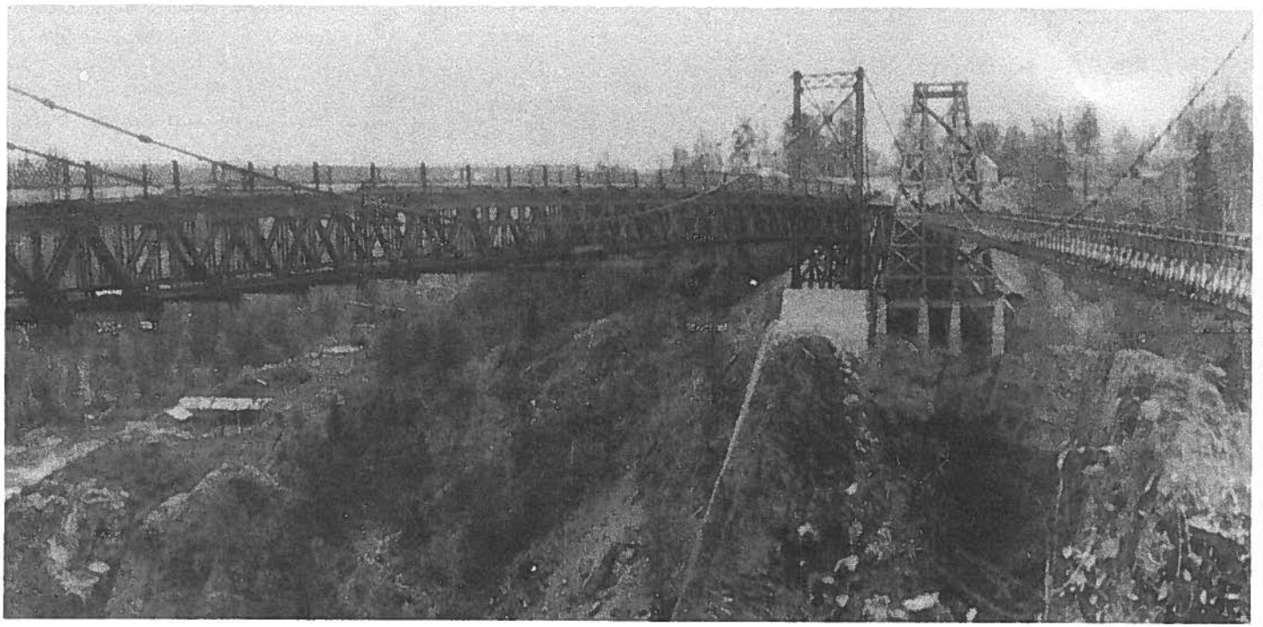
Hagwilget c. 1932. New (still existing) bridge on left, old suspension bridge (now at Walcott) on right.
