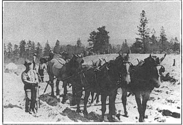
Two- and four-horse teams pulled band graders called "fresnos."
