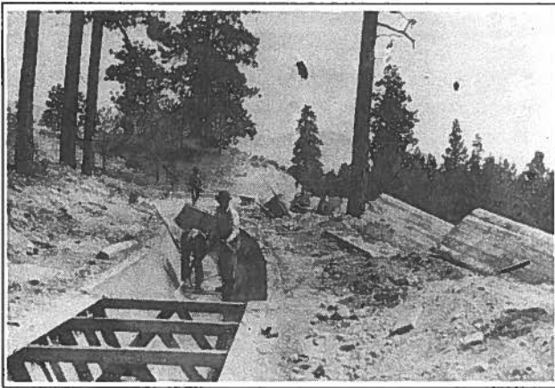
Building concrete-lined irrigation canals for the Glenmore Valley. Note the cast out forms on the right.
