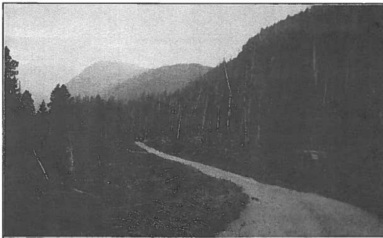
Highway 16, 1937, between Galloway Rapids & Skeena City.
