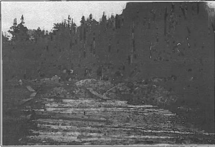
Highway 16, 1937. Corduroy road west of Prudhomme Lake.
