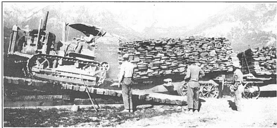
Bill Parkin on Cat 60 hauling Athey wagons loaded with snow fence up ramp beside C.P.R. siding for loading into boxcars near Fairmont Springs, B.C. Men are worried about wagon tongue. This is because an accident on a steep slope on the way in saw the front truck on the lead wagon overturn, and the kingpin dropped out. The load was taken up by chaining directly to the rear of the Cat. Athey wagons could carry 10 tons. They had a dual tracked rear wheel set.
