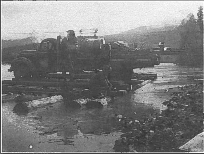
Chevrolet 'Maple Leaf' circa 1941 (Jimmy Crowe's truck). Otto Anderson on left. Raft is constructed of dry logs for better buoyancy. Rafting was necessary to retrieve 3,000 ties, equipment including a Cat, etc. on the far side of the river after the floating bridge gave way.
