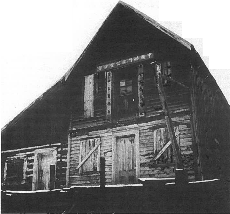
The Barkerville Chee Kung Tong building still sits in the Historic Town. This picture was taken c. 1960. Courtesy Barkerville Historic Town P639.
