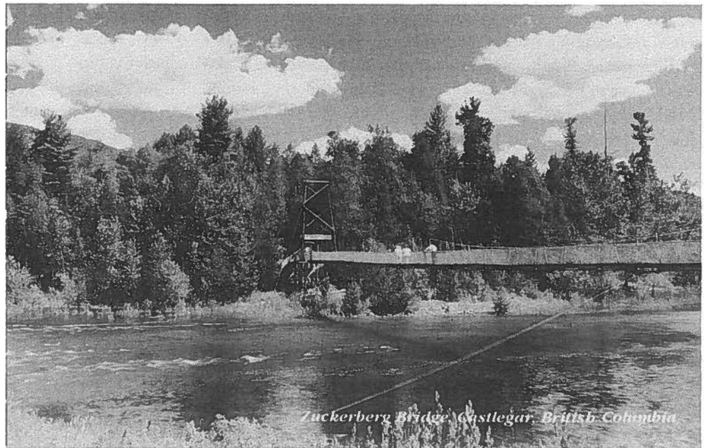
Suspension Bridge, built as a field exercise project in 1984 by the 44th Field Engineer Squadron, to connect Zuckerberg Island Heritage Park to the mainland. The 474 foot bridge was erected with donated material and won the coveted Canadian Militia Hertzberg award.
