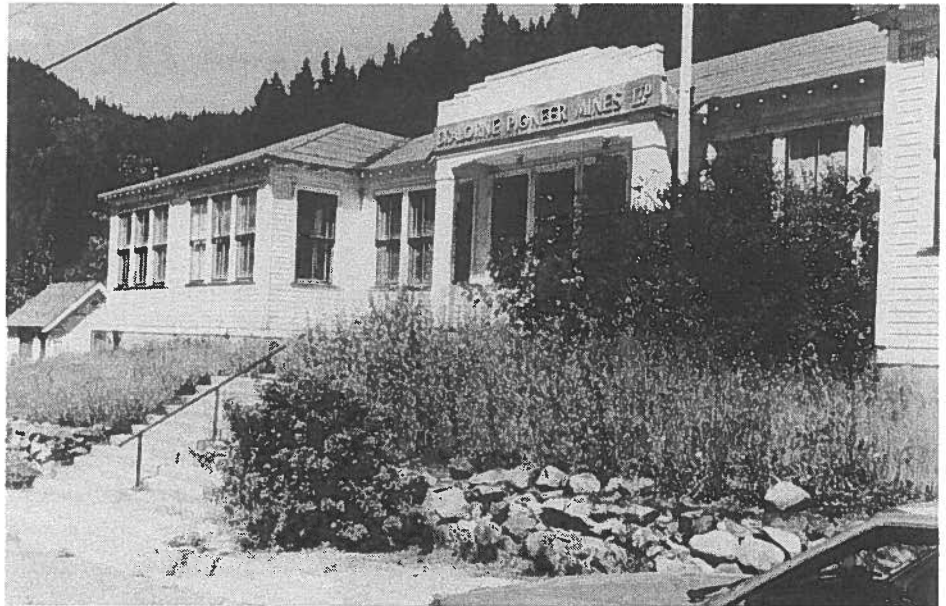
Bralorne Assay Office: recently converted into a motel.
