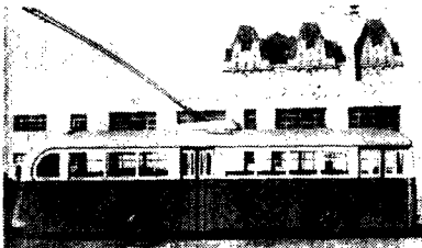
Trolley Coaches — Canadians' favourite transit vehicles—use G-E propulsion units and controls.
