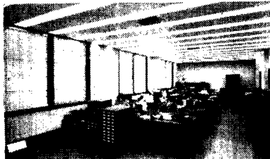
The high efficiency of electric lighting is typified by this modern G-E fluorescent installation.
