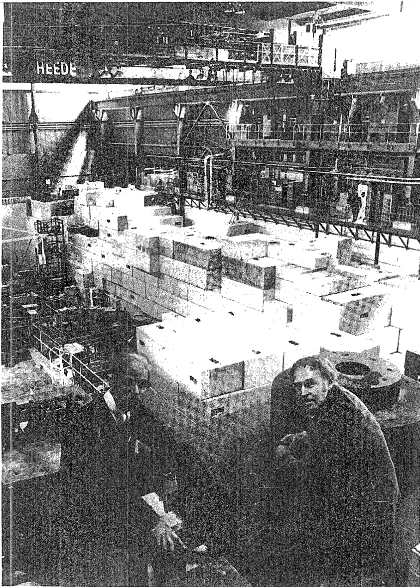
Dr. Brian Pate, left, and Joop Bergeron, senior engineer at TRIUMF, the cyclotron located on the UBC campus, are dwarfed in the immensity of the meson hall of the facility, where production of radioisotopes for use in medical diagnosis is planned. Streams of protons from the TRIUMF accelerator will pass along beam line shielded by huge concrete blocks in background and strike targets in the far corner of the building to produce radioisotopes. Picture by Jim Banham.
