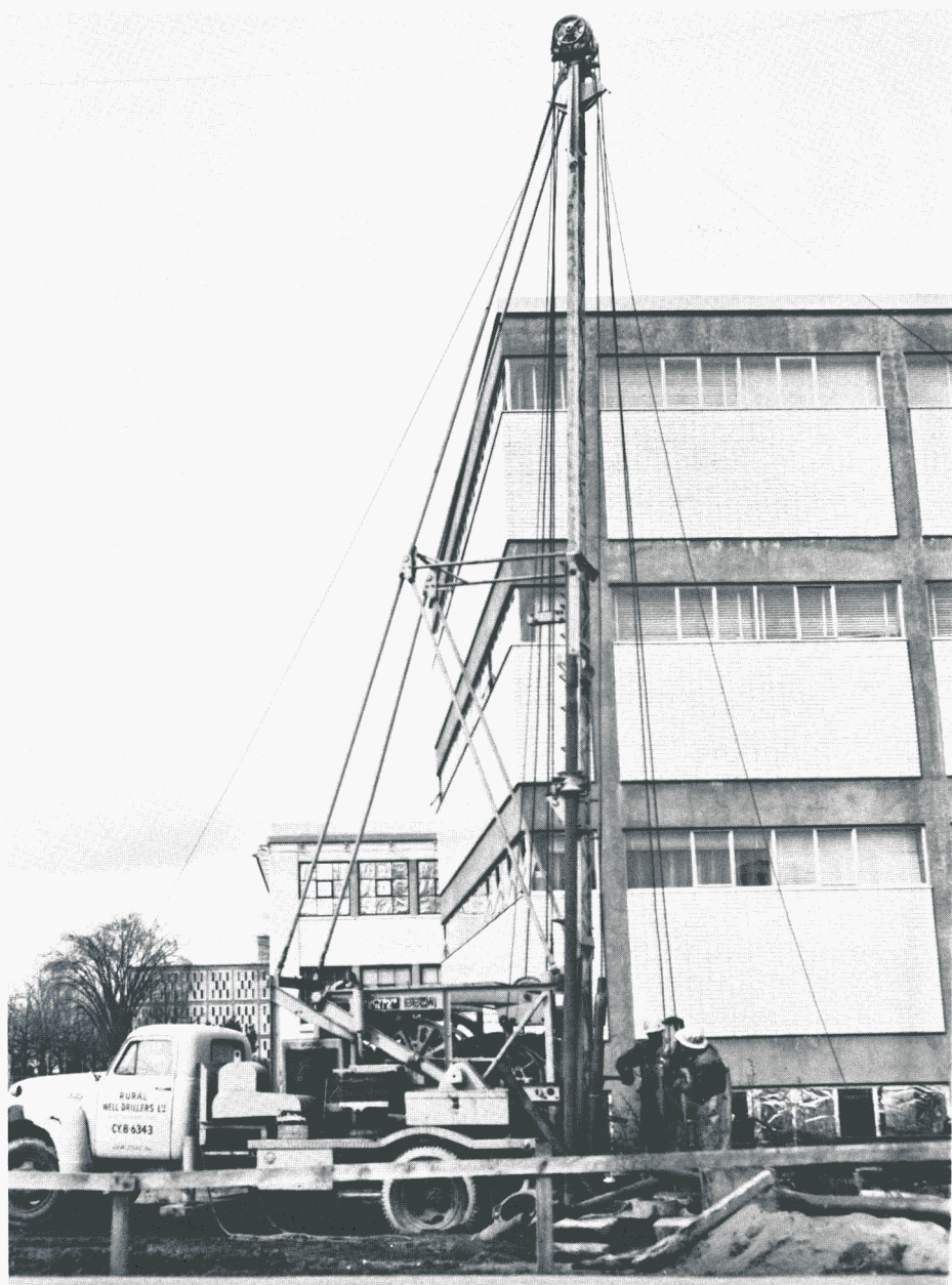
Drilling a 325-foot well at the Biological Sciences Building.
